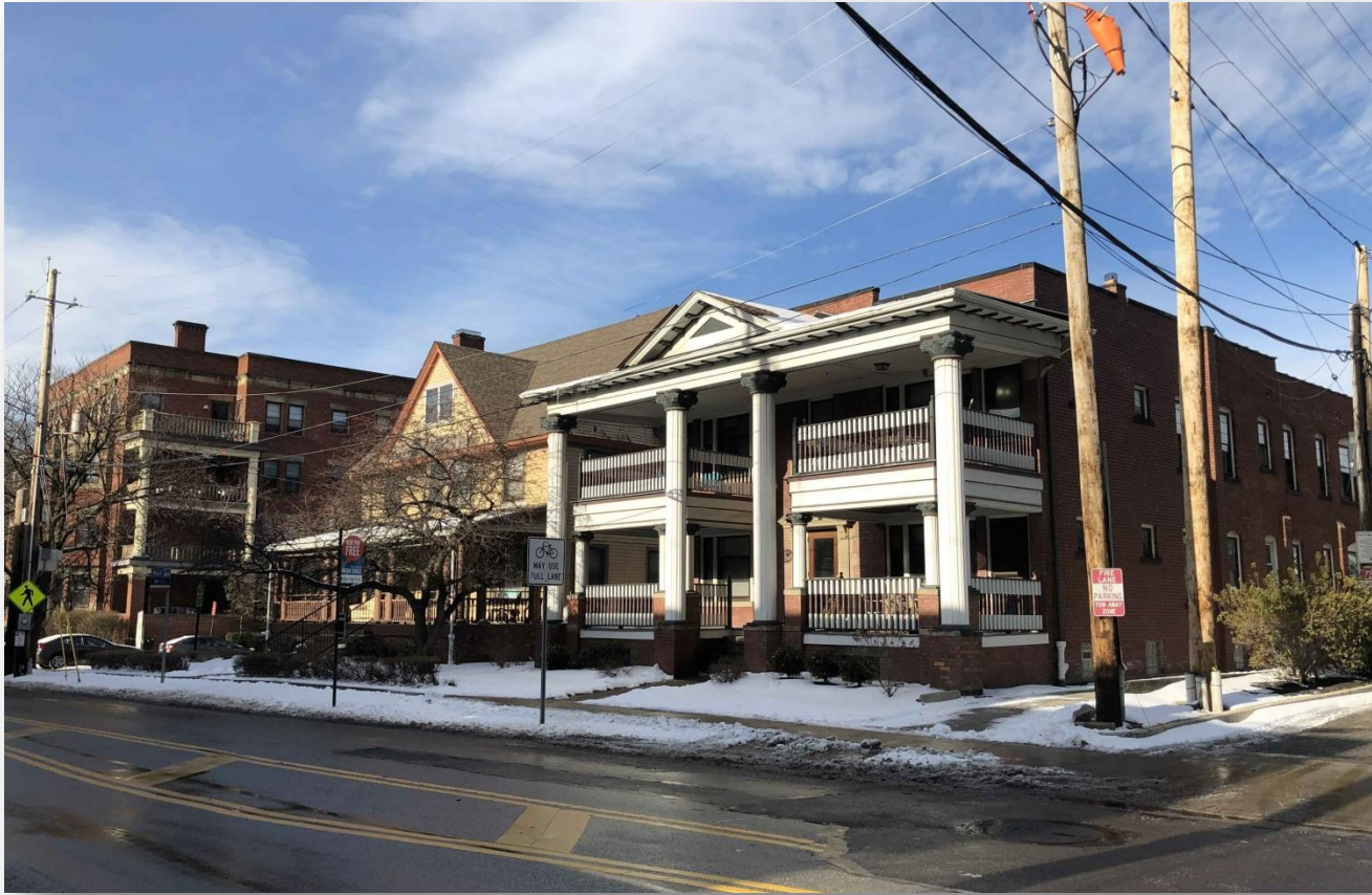
1981 Ford | Existing Apartment Building
