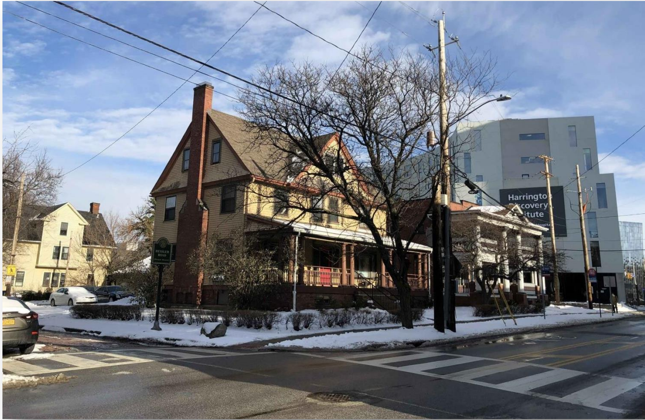
1975 Ford | Existing Apartment Building
