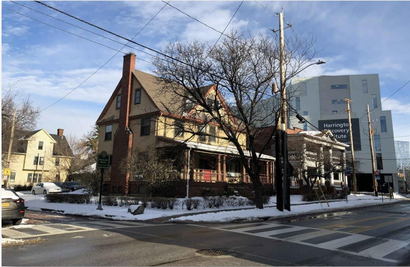
1975 Ford | Existing Apartment Building
