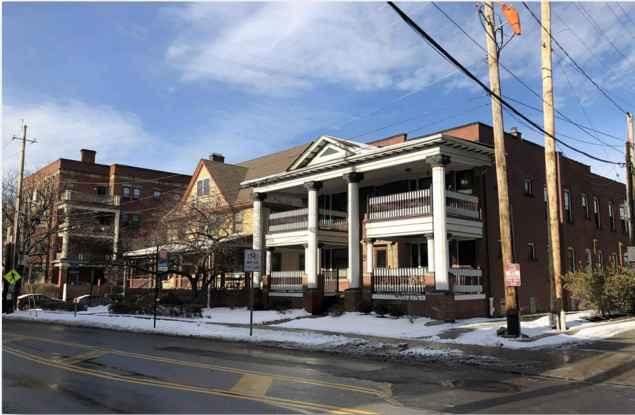
1981 Ford | Existing Apartment Building
