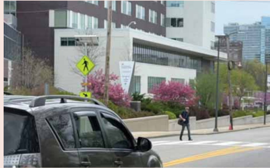
RRFB on East 105th Street adjacent to the VA
